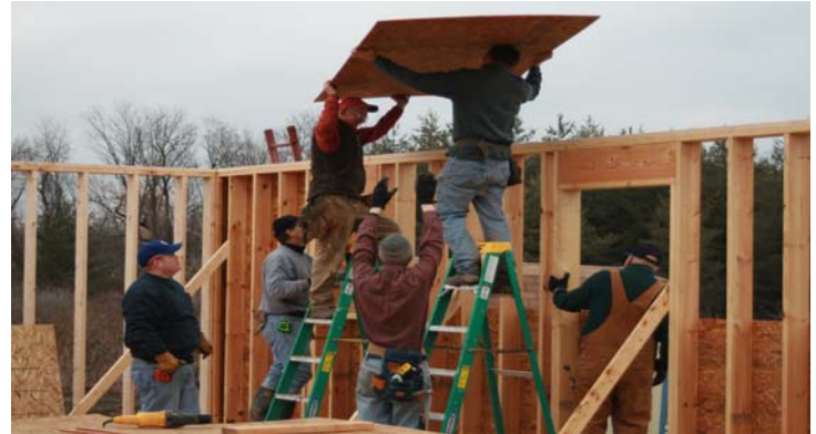
Ovid House under construction. Photo by Todd Martin
